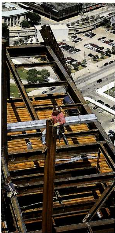
Figure 1.6 As a result of chemical change, bright steel girders become rusty when exposed to moist air.
